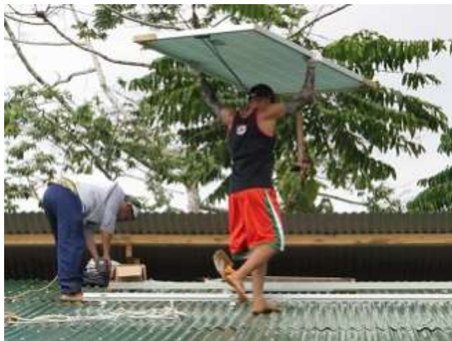
Solar panel installation in the Pangamo dalepaan
